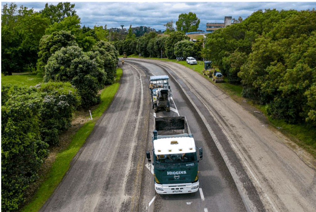
Figure 1. Pavement Sealing Work on Tennant Drive South of Massey University
