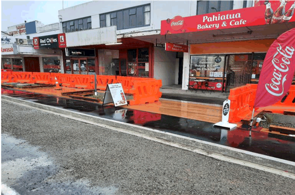
Bio-filter garden and footpaths nearing completion
